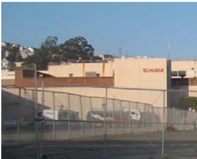
Figure 2: Schlage Lock Plant from the back.
